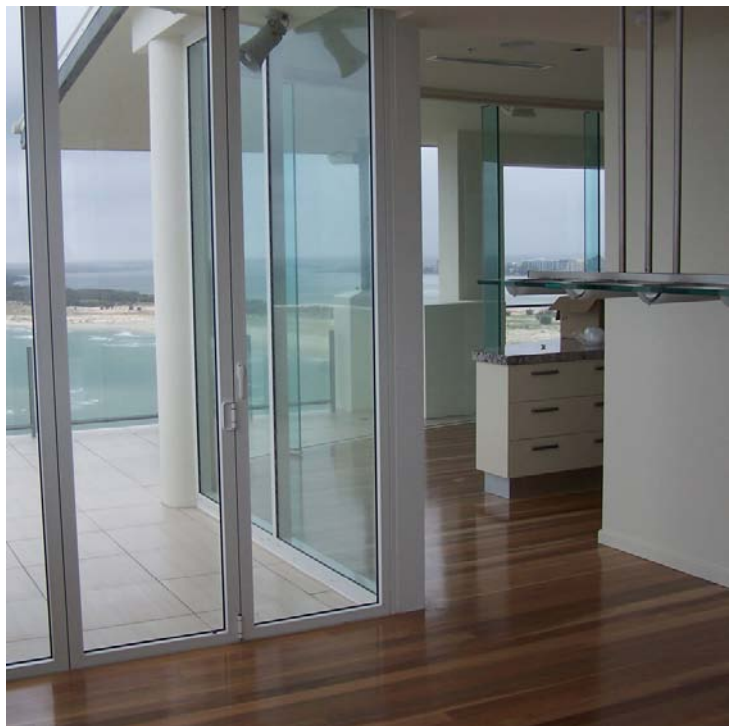
Timber floors are generally easy to maintain and greatly benefit from regular care.
